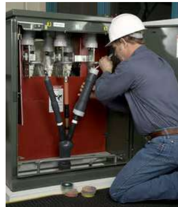
3M™ Cold Shrink QT-III Termination Kit 7600-T-3-RJS Series for 5-35 kV
